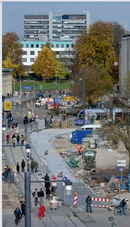
What is now a large construction site will soon be a new central square for Freiburg. Photo: Thomas Kunz
